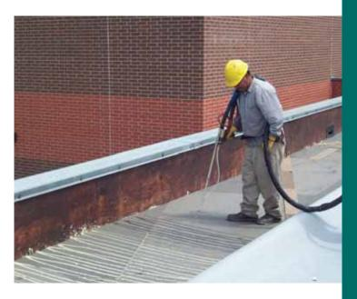
puncture resistance and 33% greater breaking strength than standard 60-mil TPO. Crawford believed it was the ideal choice for the district's need due to its superior hail damage resistance—the membrane passes FM's severe hail test and the National Bureau of Standards ice ball test for hail up to three-inch diameter with the membrane cooled to 32°F. It also holds a UL-2218 Class 4 rating.
